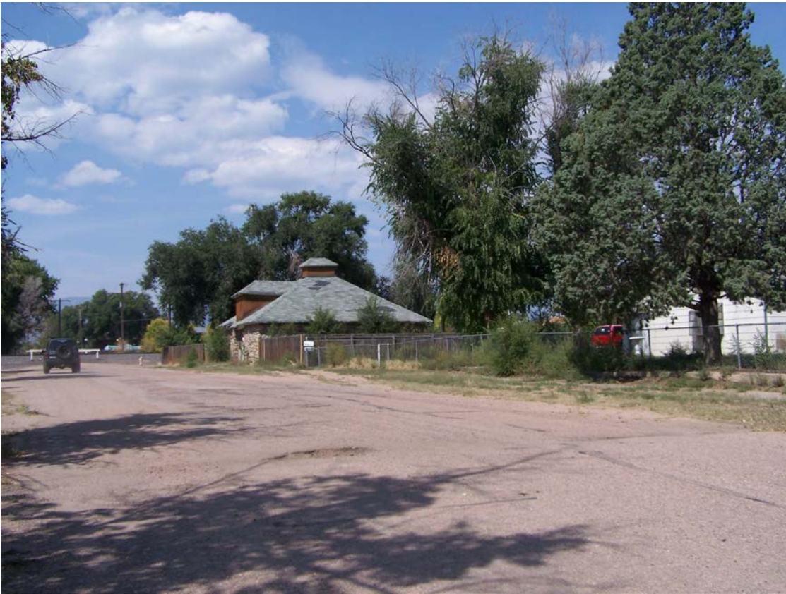
Nationally Designated Historic "Livery Stable" Site – deteriorating roof structure
