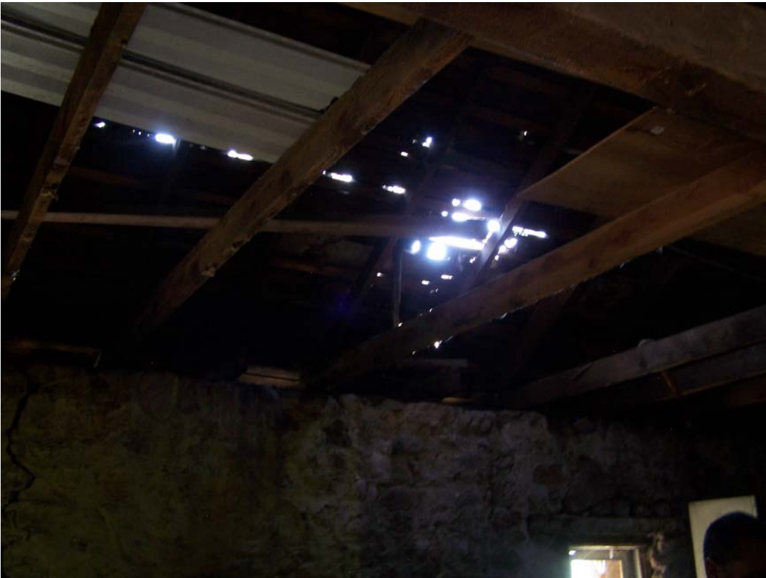
Nationally Designated Historic "Livery Stable" Site – rock wall structure
