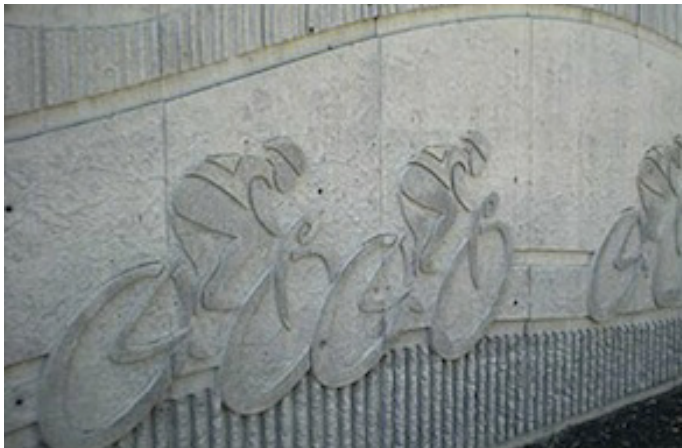
Example: Formliners can be customized to create texture and pattern
