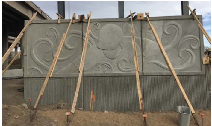
I-25/Ilex: Form liner panels developed for I-25 abutment walls at Ruynon Field
