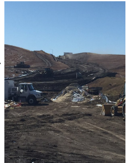
Venetucci Blvd. grading and earthwork
