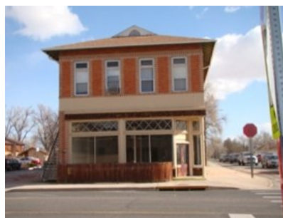
Woodman Hall frontage on Main Street
