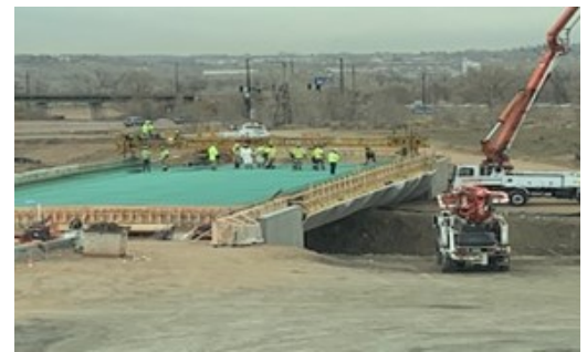
Venetucci Blvd. bridge girders and caissons
